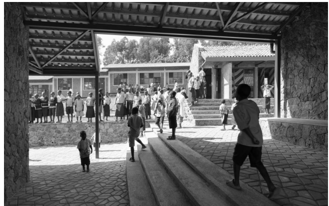
Figure 5. Ruhehe Primary School, Ruhehe, Musanze District, Rwanda: 2018. https://massdesigngroup.org/work/design/ruhehe-primary-school .
